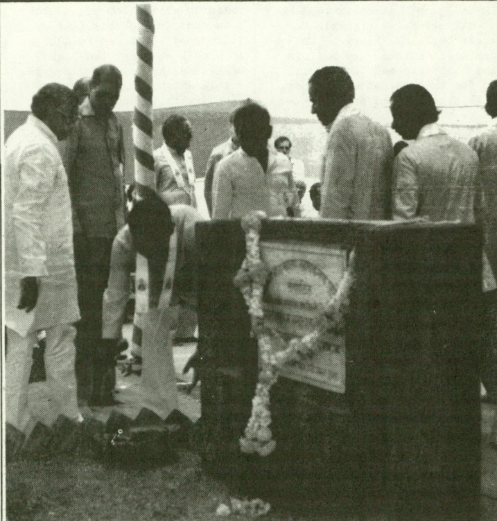
Laying the foundation stone at Dapodi
